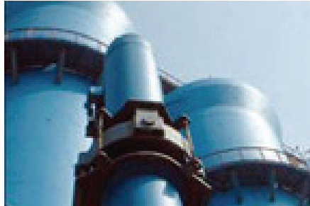
Fig. 6. Blast furnace hot stoves, the large heat exchangers for heating the air-blast to over 1000°C prior to injection into the blast furnace tuyères.
