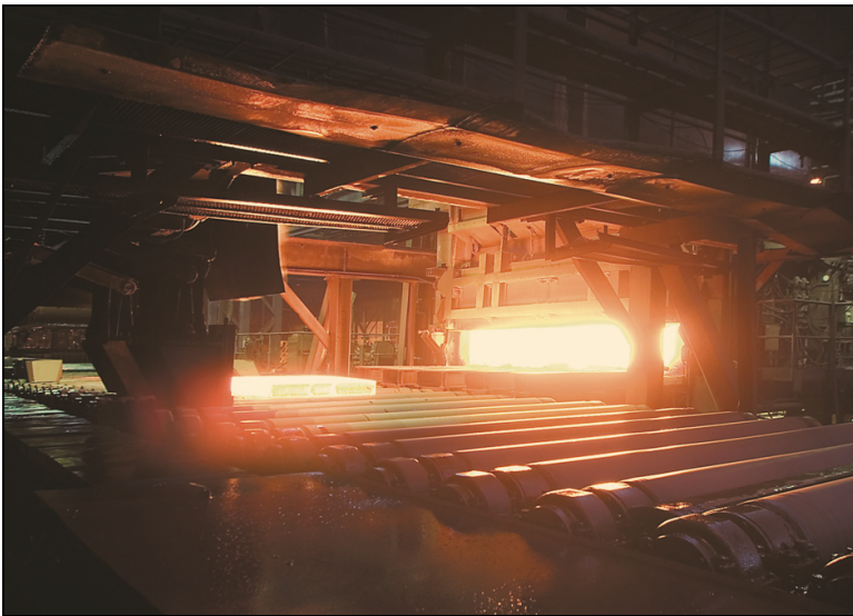
Fig. 9. A heated slab is discharged from the walking beam furnace at Outokumpu's Degerfors Works. Here flameless oxyfuel has increased the heating capacity by 40-50%.
